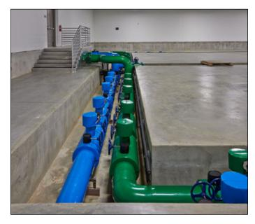
No shared infrastructure, chilled water loop sized for expanded critical load
